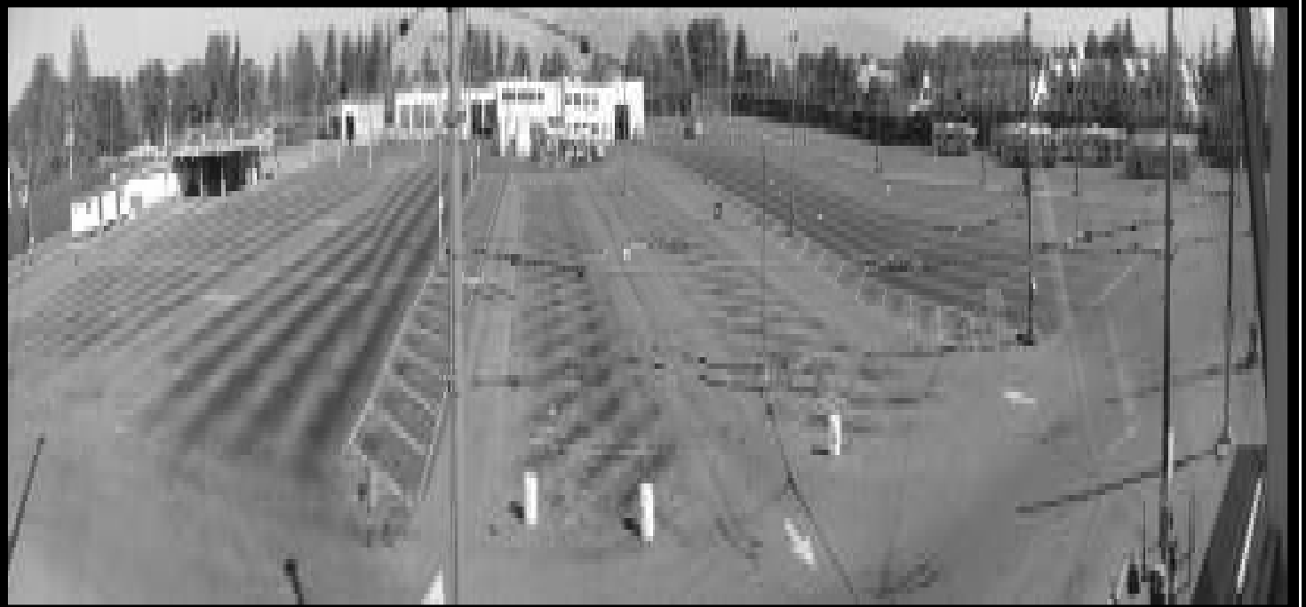
Empty OTC from the Control Room
